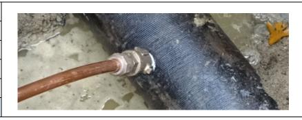
It has been discovered that when the new waterline main in Weld County Road 21 was installed, the existing service lines were not moved to this new main. These services must be moved to allow shut down of the old ductile metal waterline in Weld County Road 21.
